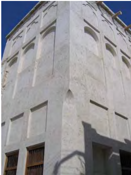
Exterior being renovated in Muharraq
