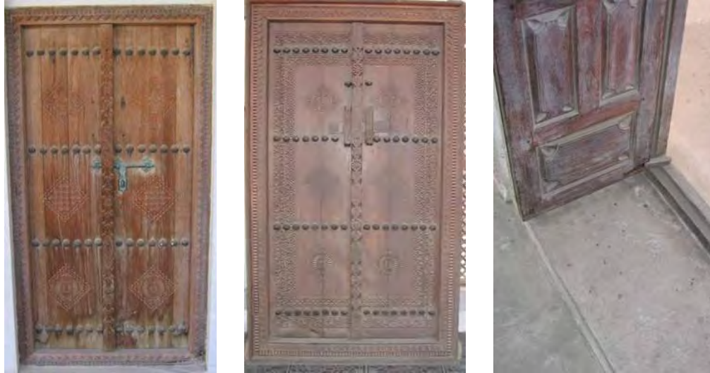
Left: old door after conservation, middle: new door made according to traditional design. The two in the house of Salman in Manama. Left: wooden peg to keep door open at House of Bin 'Issa in Muharraq.
