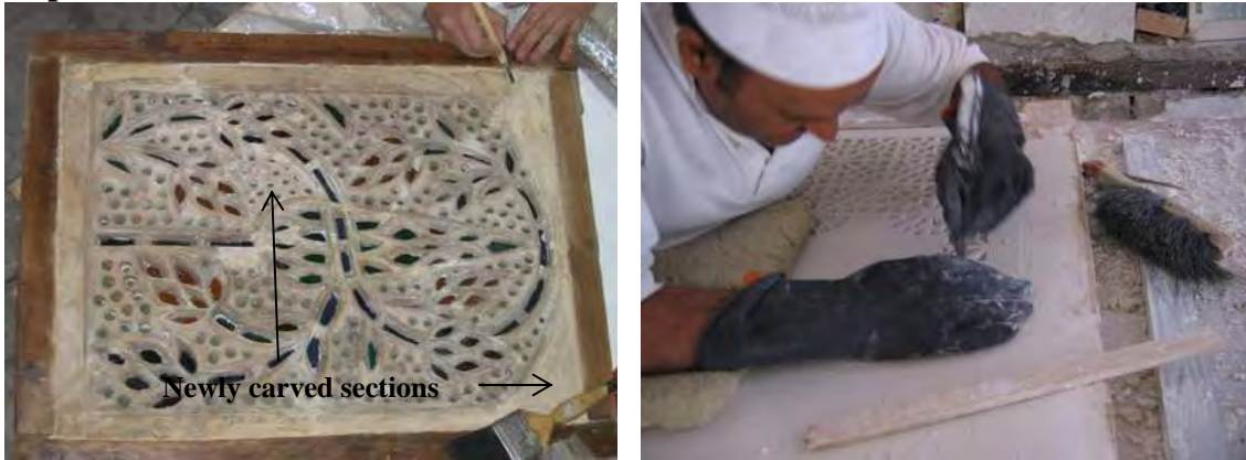
Left: old gypsum window restored by preserving its pieces; Right: Nagui carving a new gypsum window.
