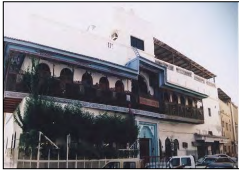
Metal Roof Structures Spoil Appearance
