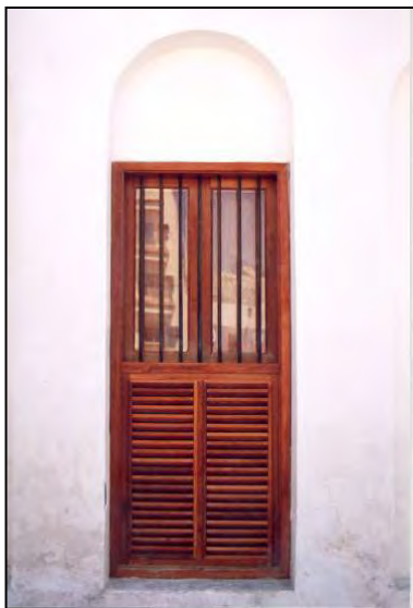
IRON WORK COMBINED WITH TIMBER SHUTTER
