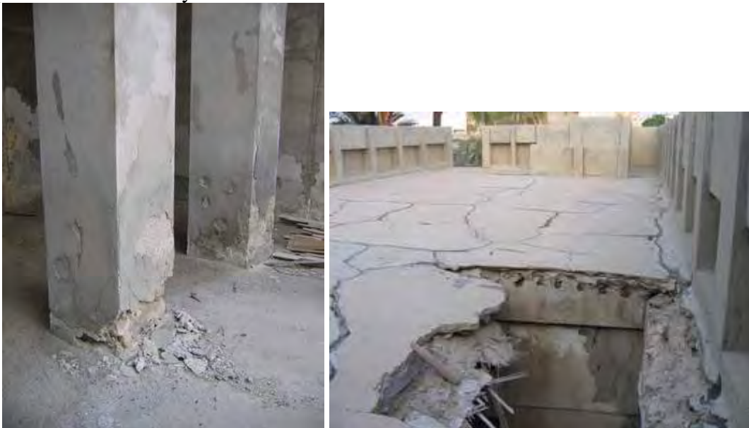
Cement plaster over vertical architectural surfaces in the house of Shaykh Salman House in Muharraq
