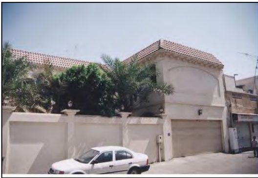
DOUBLE WIDTH DOOR PROHIBITED
