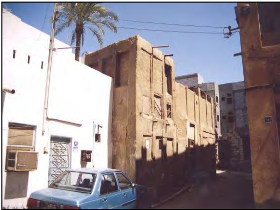
Typical Fabric Buildings
