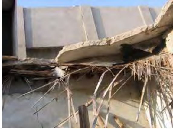
Roof failure in house of Shaykh Salman, Muharraq
