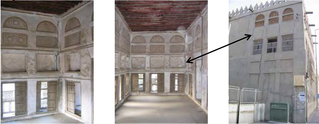
Sheikh Salman House: first floor room. Note the corner longitudinal crack. Note the external network of continuous longitudinal cracks developed due to foundations' differential movement.
