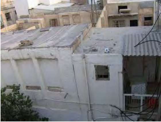
Roof of House of Jasim al-Qusayr in Manama
