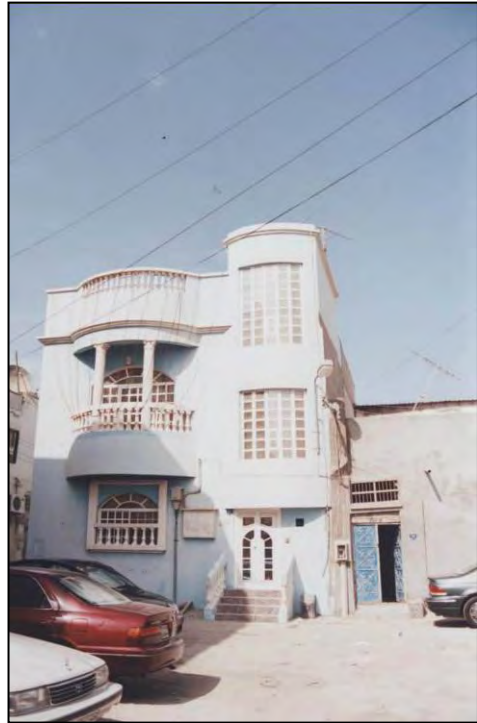
Inappropriate Architectural Style
