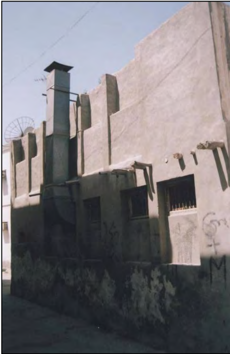
Improper Mechanical Interventions
