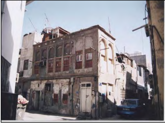
Typical Fabric Buildings
