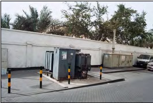
SCREENS ERECTED AROUND UTILITY INSTALLATION
