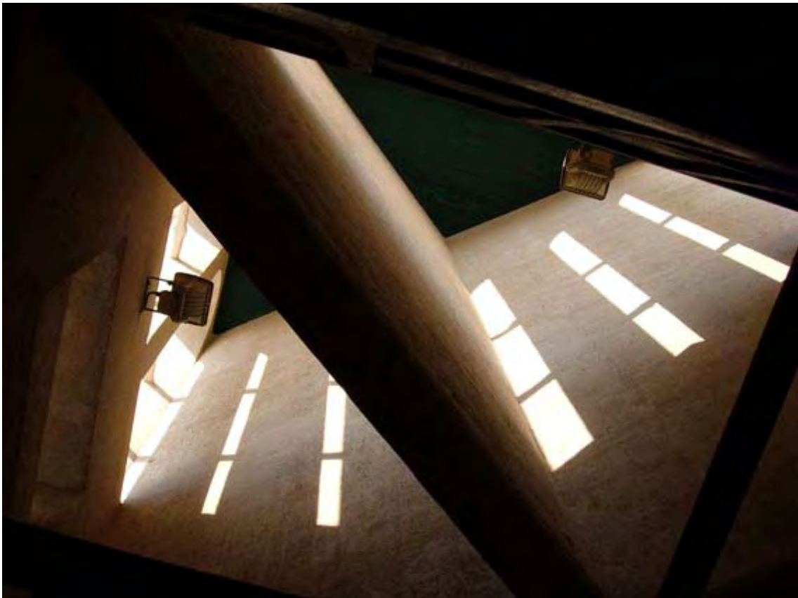
Photograph looking up into the wind tower of Shaikh Isa Ibn Ali Al-Khalifa House
