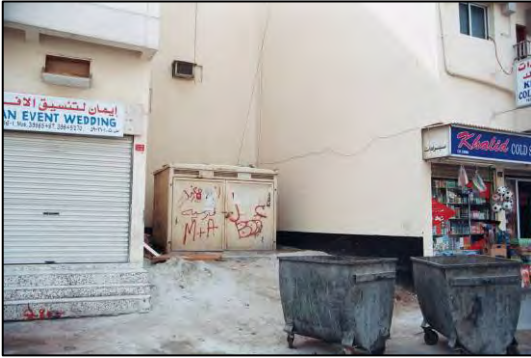
EXISTING UTILITY INSTALLATION BETWEEN TWO BUILDINGS: ADD SCREENS MIN. 3M. HIGH
