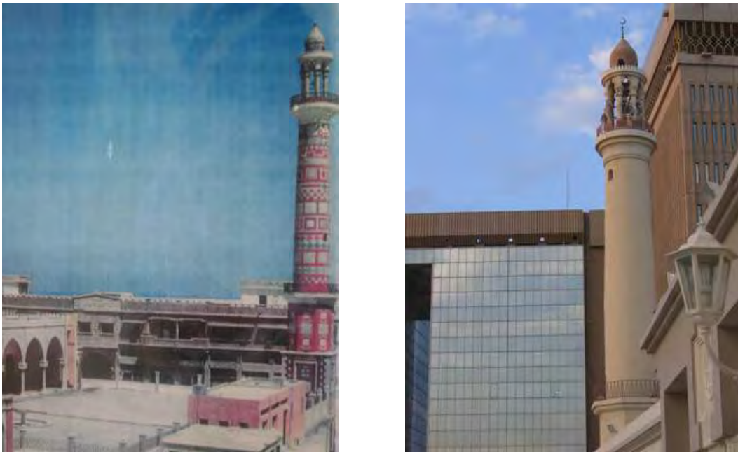
Minaret of the Mosque of al-Fadil before and after intervention. No attempt to indicate historic layering.
