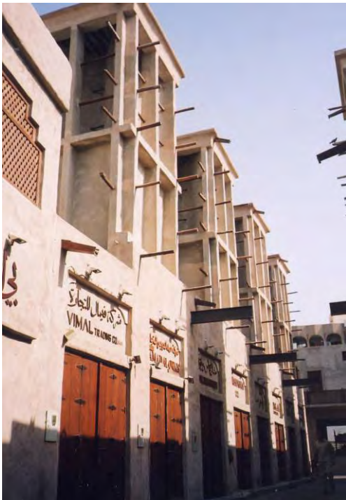
FRONT LIT SURFACE MOUNTED SIGNS
