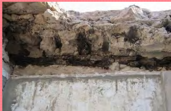
Denchel wood eaten away in Shaeih Salman house caused the collapse of the floor
