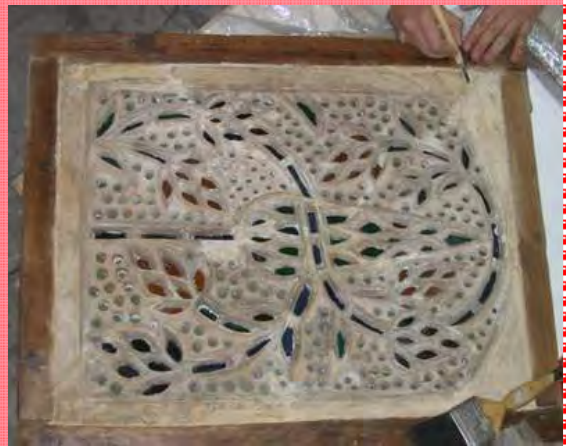
Old gypsum window restored by preserving its pieces;
